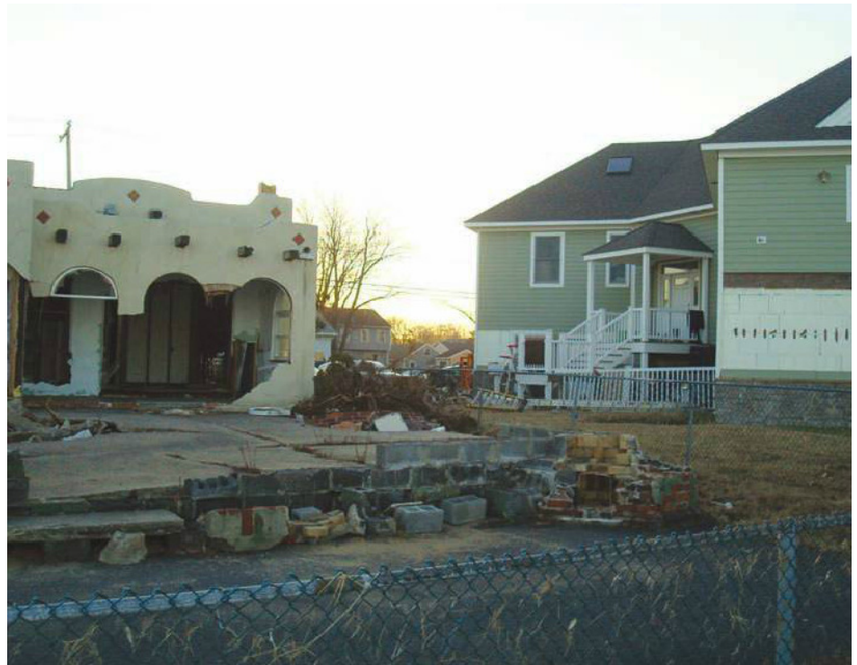
The Hallet house lost some exterior siding, and some damp drywall will have to be replaced. That's the full extent of damages.
